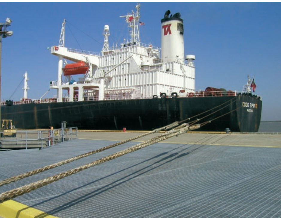
Rodeo Terminal upgrade California, USA.
