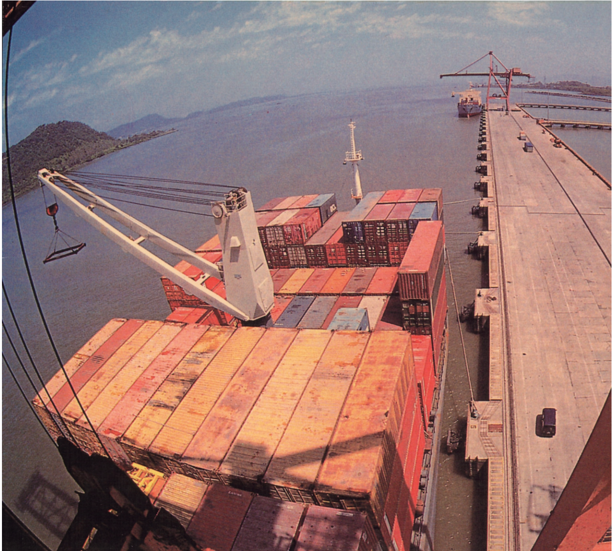
Bird's-eye view of the existing port of Jawaharlal.
